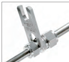
Properly tightened, the gauge will not fit
